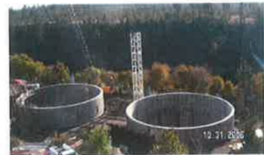
Tower crane assembly.
