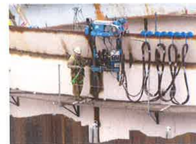
Horizontal welding process on side of digester.
