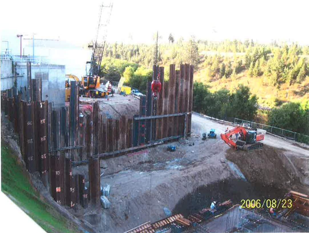
Exhibit C: Shoring east area of site, looking southeast.
