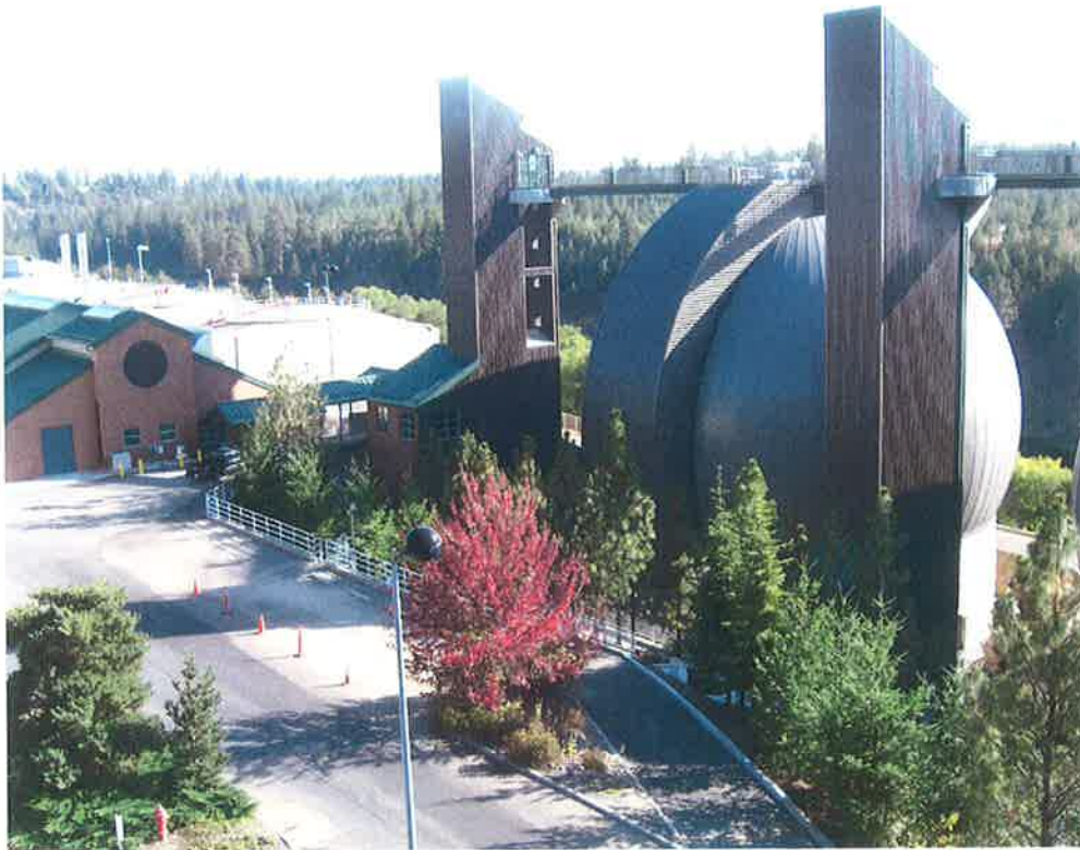
Exhibit L: Digester and boiler building.
