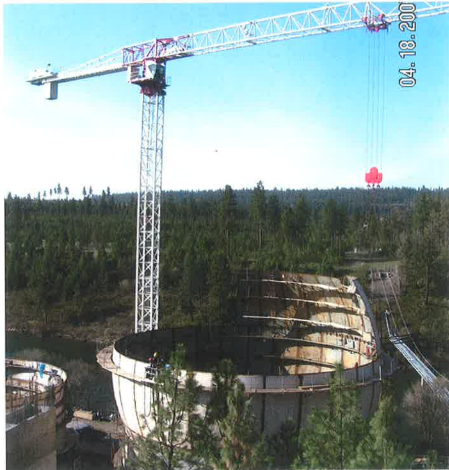
Exhibit F: Setting tank wall section (note scaffolding in place).
