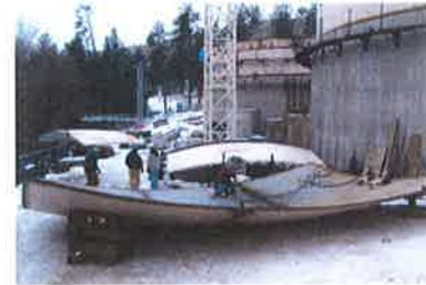
Welding tank panels on ground between digesters and river.
