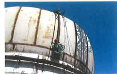
Vertical welding process on side of digester.
