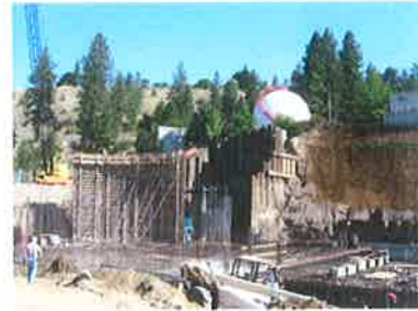
View from foundation level, looking up hill.
