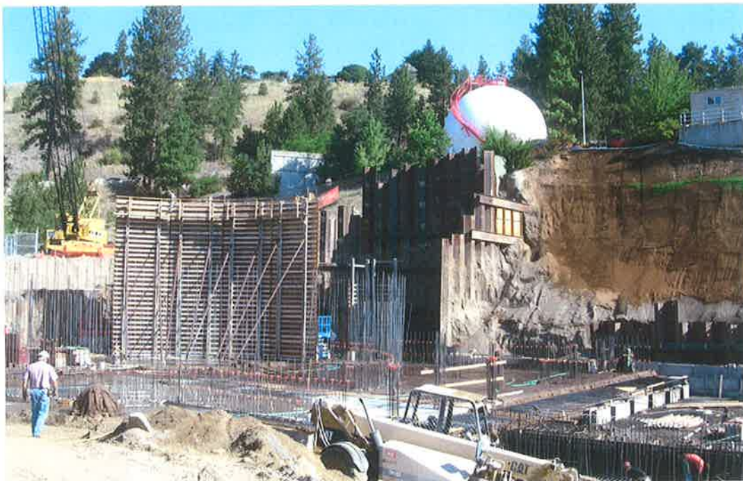
Exhibit B: View from foundation level looking uphill.
