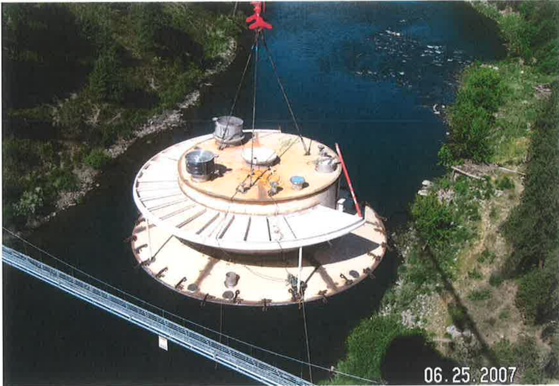
Exhibit G: "Flying" digester dome lifted in place over Spokane River.
