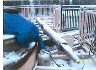
Top of Digester 4, looking north, with steam lance nozzle.
