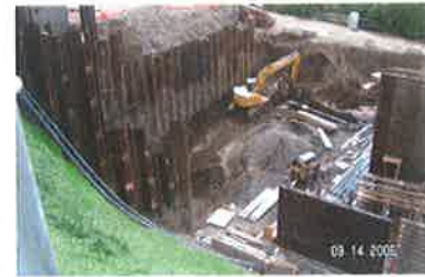
Sheetpiling and excavation adjacent to Digester 3 and existing digester building
