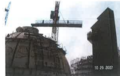
Selling digester bridge.
