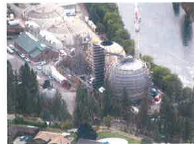
View of project from neighborhood above facility.
