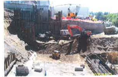
Eastside shoring and excavation with foundation progressing from west.
