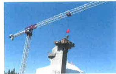
Stair tower construction.
