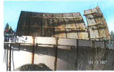
Selling tank section with scaffold.
